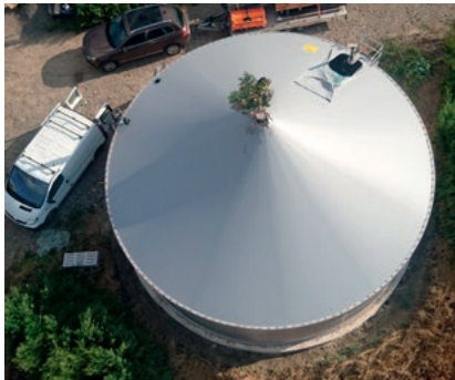
Membrandach von oben | Membrane roof from above
